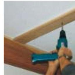
An EZ BEAM ceiling can be laid out in proportion to the custom specifications of any room. Beam sides differ in height, the tallest trimming the perimeter of the room, the shorter providing the main beam structure running the length of the room, the smallest serving as the cross-members between the main beams.
