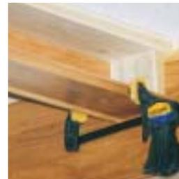
Repeat procedure to attach opposing side-member. Continue until all beam sides and bottoms have been positioned and nailed. Install bed moulding around the top, inside corner of the square formed by the installed beams.
