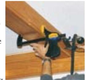
Attach beam side to blocking. The nails securing the side to the blocking will be covered later with bed moulding. Fit the bottom component into the side-member groove and clamp into position. Nail side-member to beam bottom through nailing groove.
